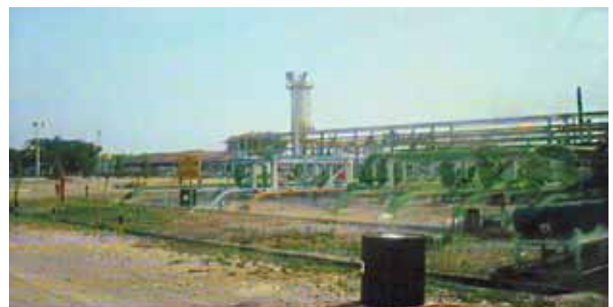
Figure 5. Modern Oil Production from Mudi Field. (JOB Pertamina – Petrochina East Java).
